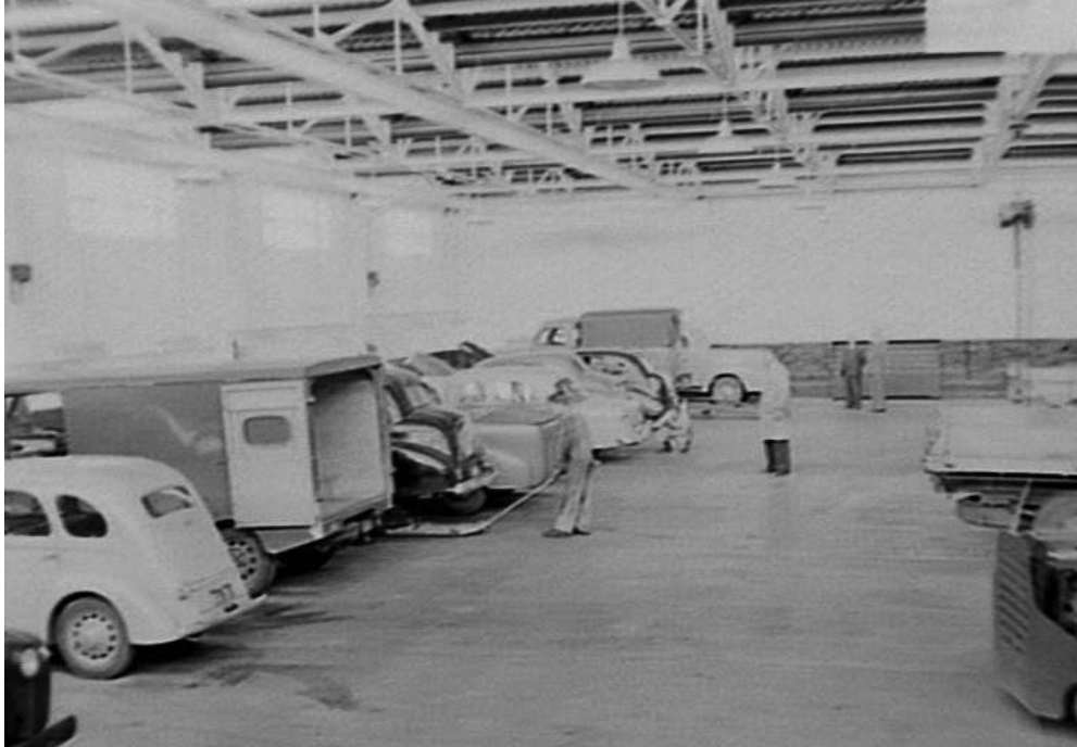
Figure 2.31 The servicing area of the 1947 garage extension
